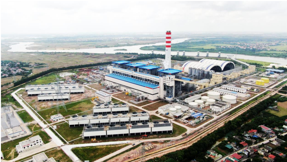
Overview of Jaks Hai Duong power plant
